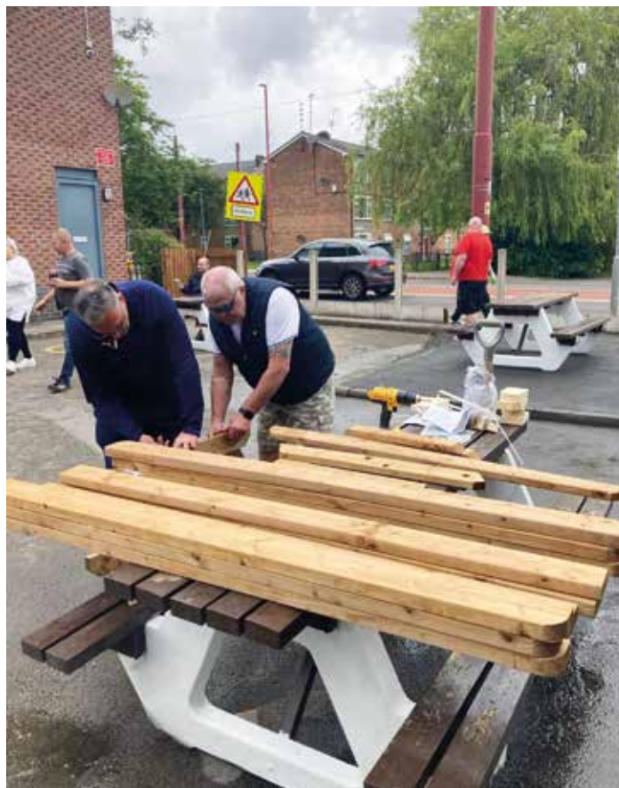
Pictures from the refurbishment and the finished project.
